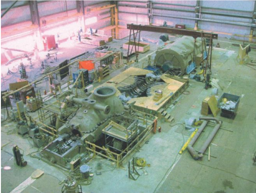
TURBINE GENERATOR CONSTRUCTION
